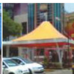
Textile Architecture Structures
